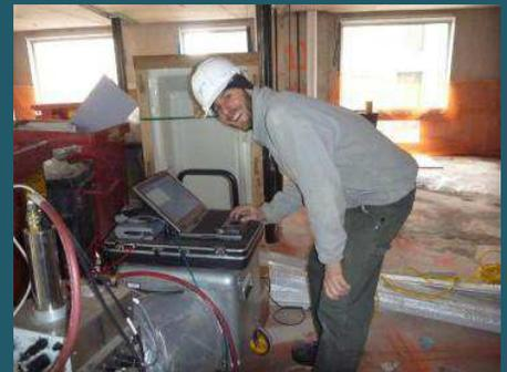
*Evan Hallas measures duct leakage in a 20-story apartment building in NYC.*
