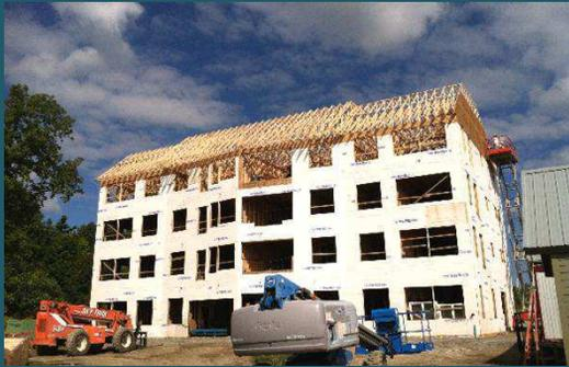
Taitem is hard at work on the new TREE neighborhood at EcoVillage Ithaca. There are four floors in the common building, and the **framing of the third floor is complete.**
