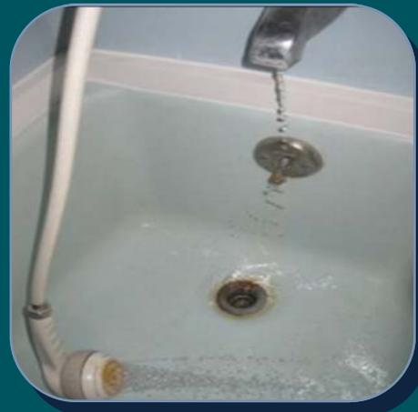
**A leaking diverter allows water to flow out both the showerhead and the tub spout simultaneously.**
