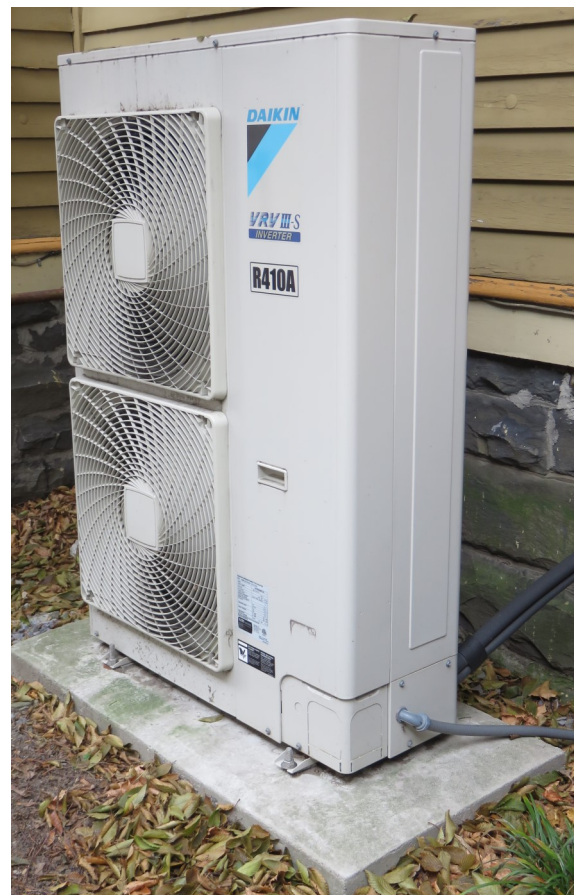
ASHP outdoor unit
