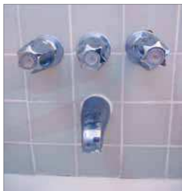
This diverter valve is part of a three-handle shower valve.
