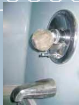
Some examples of plate diverters. Left to right: a lift on the tub spout diverter with a two-handle valve; a pull-down ring on the tub spout diverter with a single-handle valve; and a button on the valve plate with a single-handle valve.
