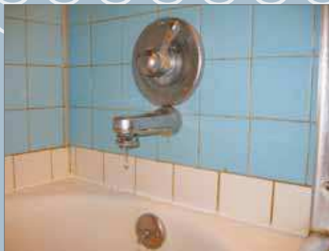
Some examples of plate diverters. Left to right: a lift on the tub spout diverter with a two-handle valve; a pull-down ring on the tub spout diverter with a single-handle valve; and a button on the valve plate with a single-handle valve.
