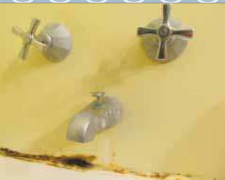
Some examples of plate diverters. Left to right: a lift on the tub spout diverter with a two-handle valve; a pull-down ring on the tub spout diverter with a single-handle valve; and a button on the valve plate with a single-handle valve.
