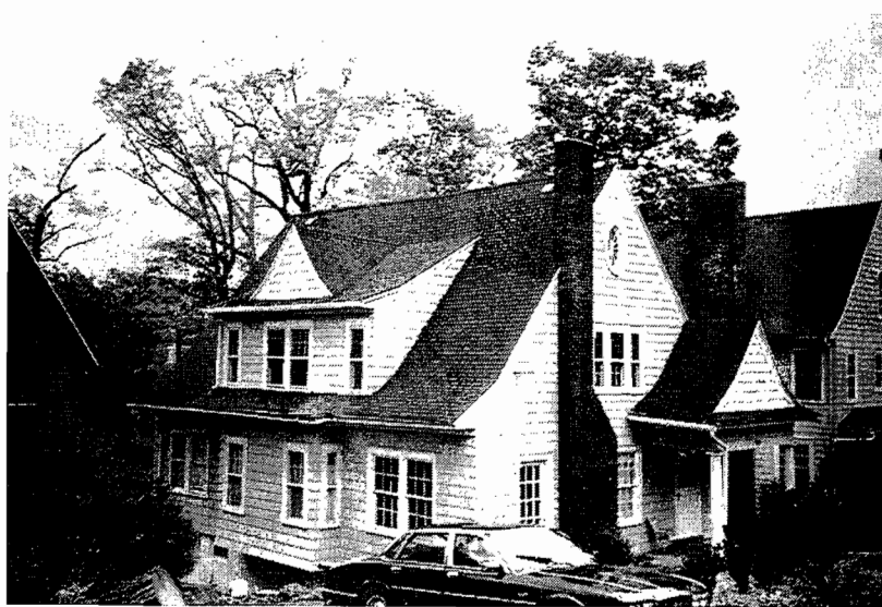
Plate 1. View of the test house from the Southeast.
