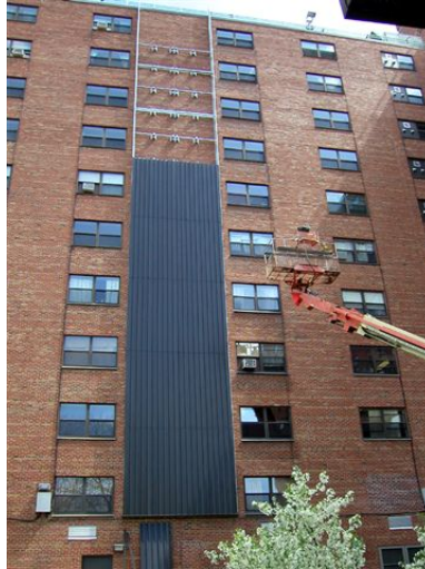
Installing the cladding
