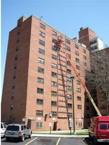
Installing the framing
