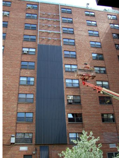
Installing the cladding
