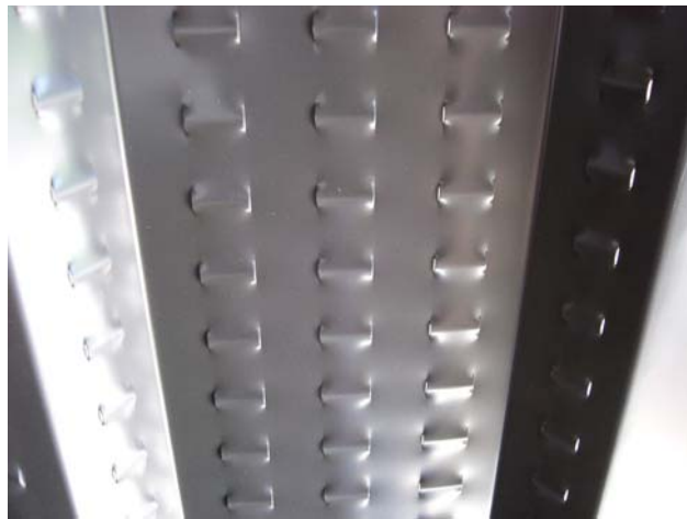
Figure 2: Close-up of Solar Preheater Cladding (Photo: Taitem Engineering)
