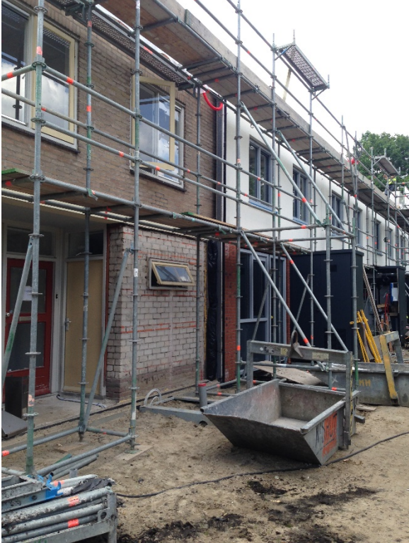
Figure A15. A closer look at the existing façade and scaffolding for renovation
