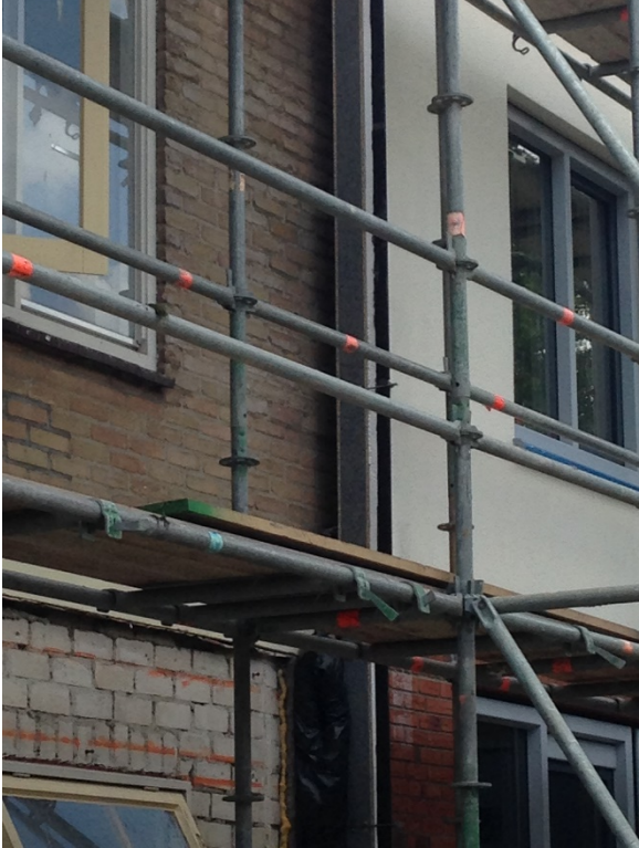
Figure A16. New exterior wall assembly seen over the existing wall
