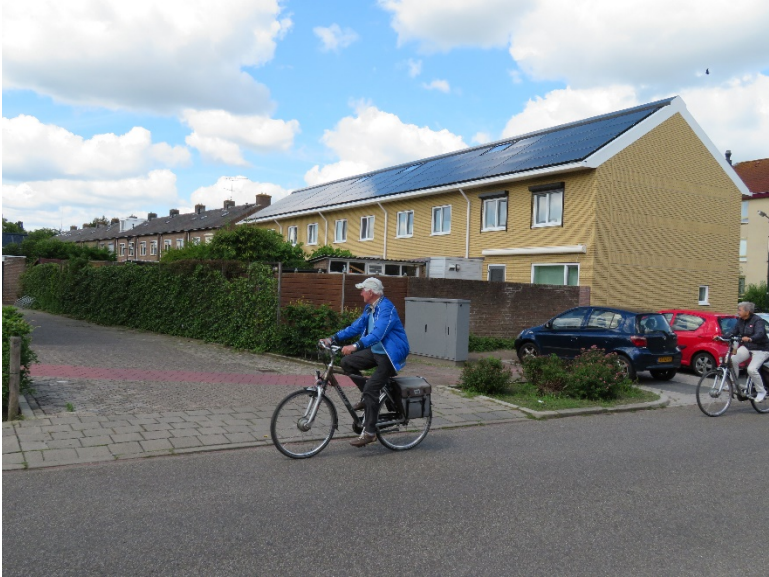
Figure A44. Renovated building
