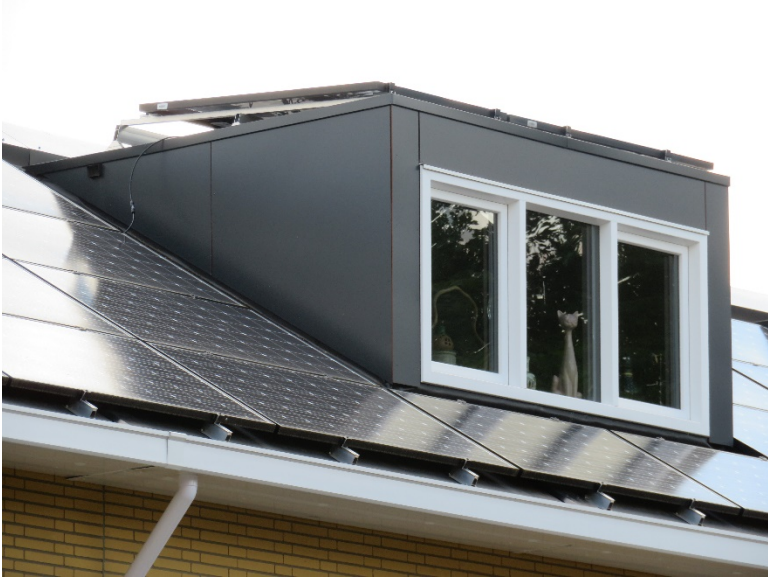
Figure A42. Dormer in renovated building
