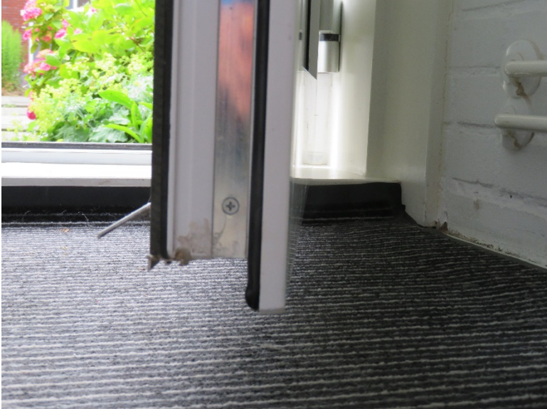
Figure 17. The doors are high-performance gasketed and insulated doors
