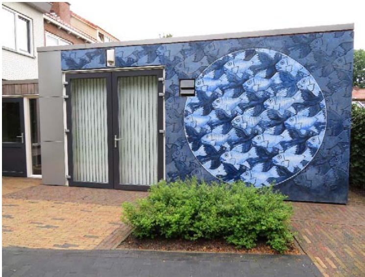
Figure 31. First floor “age-in-place” addition
