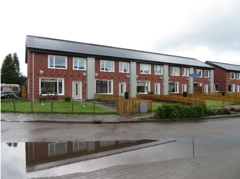
Figure A20. Renovated building with shallow mechanical chase and individual exhaust fans
