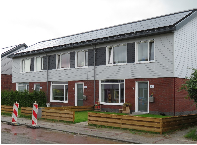
Figure A21. Renovated building (second contractor) with mechanical addition in the rear
