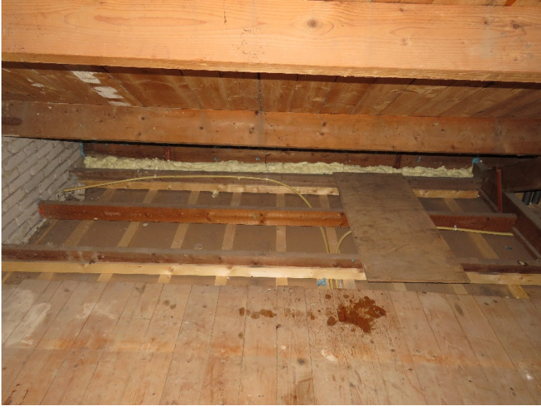
Figure A36: Attic in renovated building showing evidence of air sealing, but the insulation is all exterior, above the roof-line
