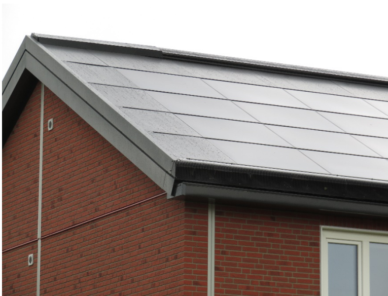
Figure 27. Roof-mounted heat pump heat exchanger: air grilles are above gutters and at roof peak
