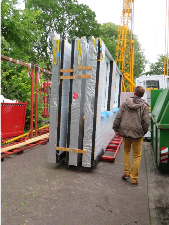
Figure 10. New wall cladding sections are brought on-site by truck
