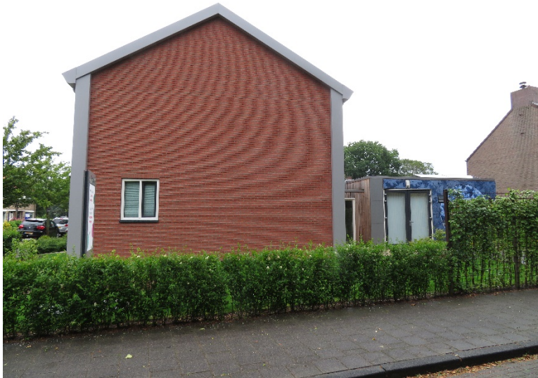
Figure A 37: Gable end of renovated building, with age-in-place addition shown at right
