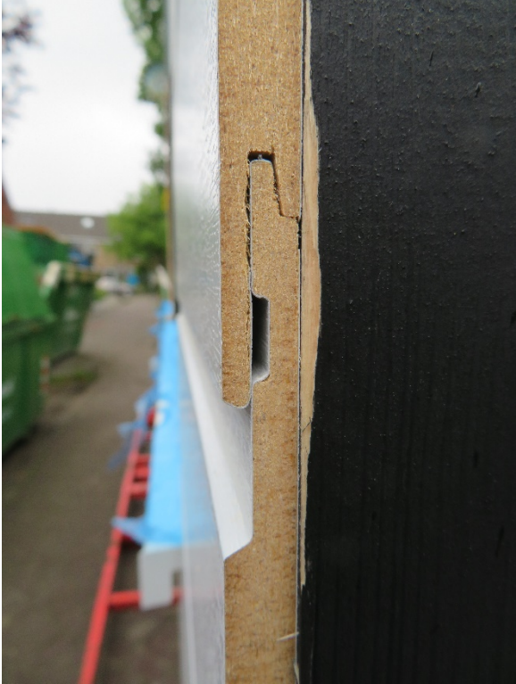
Figure 14. Alternative siding includes particle-wood with a protective facing
