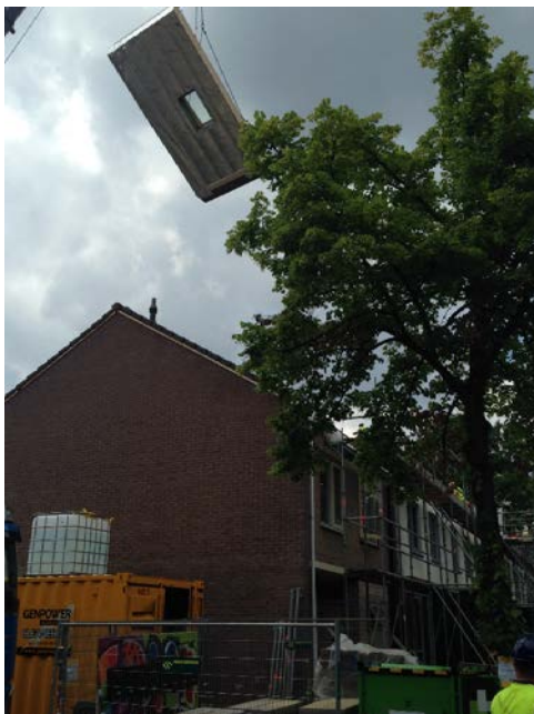
Figure 19. Roof sections are lifted by a crane
