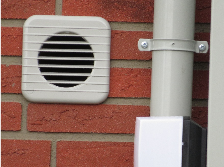
Figure 28. Room by room ventilation
