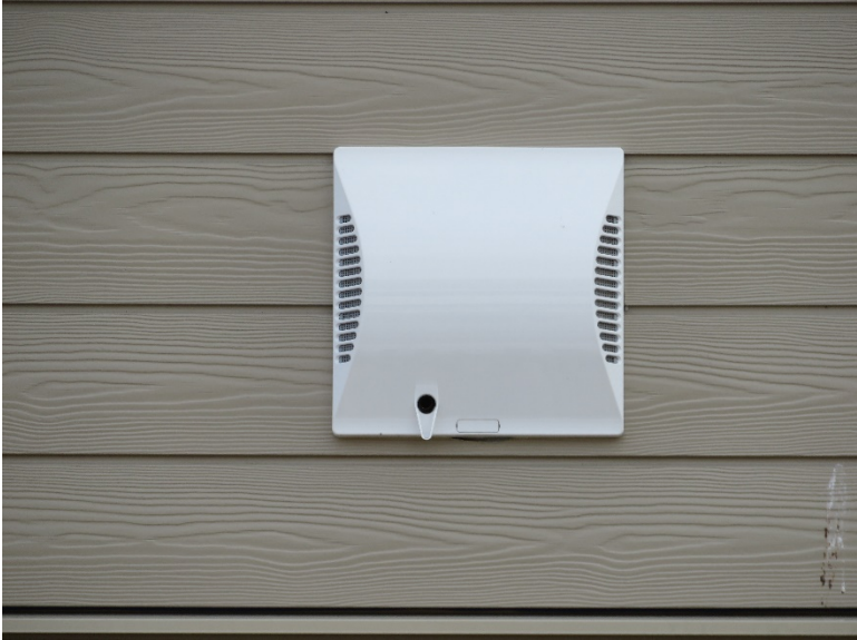
Figure A50. New ventilation fan used on a room-by-room basis
