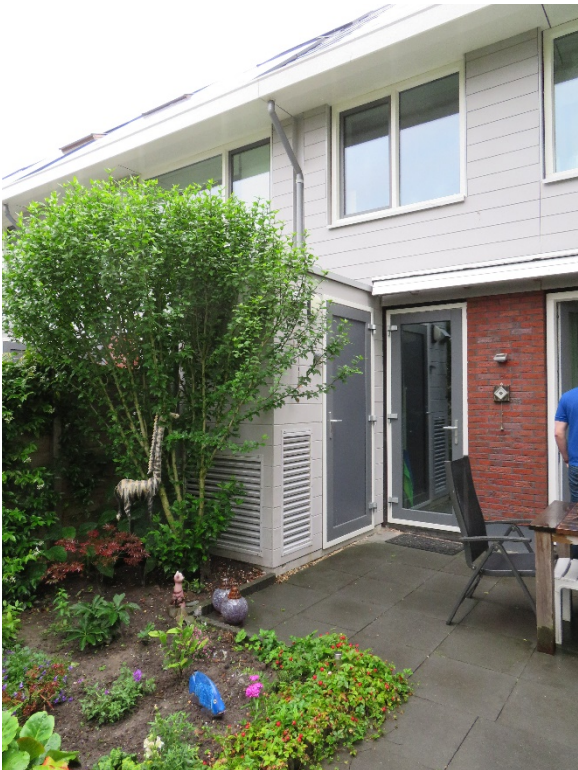
Figure A3. Mechanical rooms are in the rear
