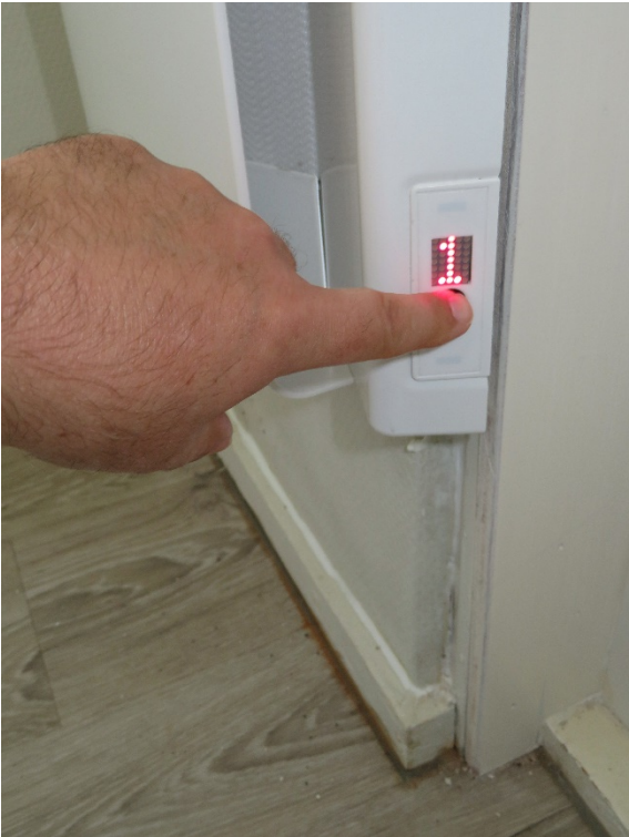
Figure A52. New ventilation fan used on a room-by-room basis
