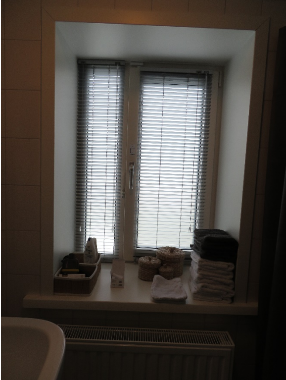
Figure A33. New windows, with extension showing depth of wall.
