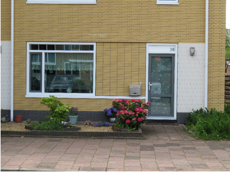
Figure A41. Renovated façade
