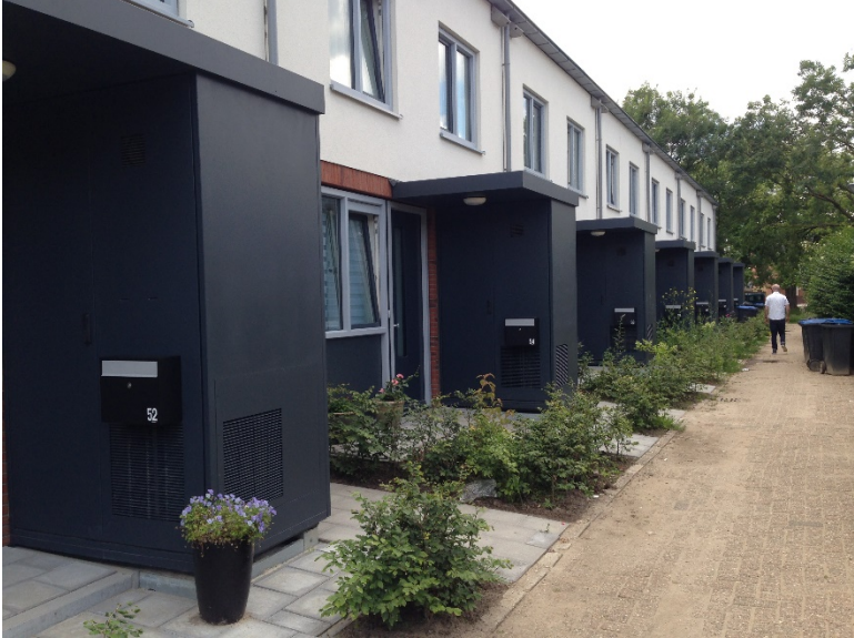
Figure A11. Mechanical rooms are in the front of the buildings
