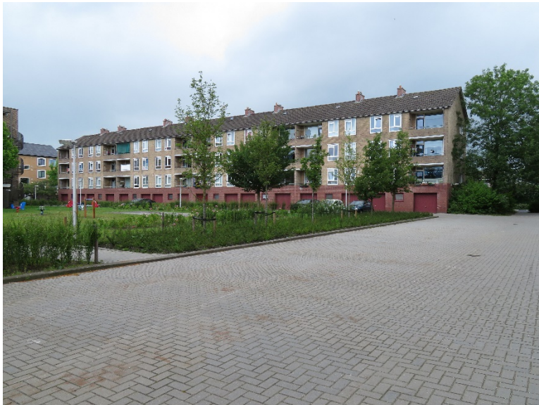
Figure A22. Building not yet renovated
