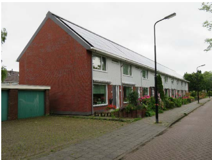
Figure A2. Renovated building
