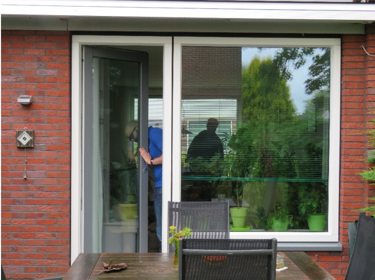
Figure A7. Exterior patio – new rear window and door
