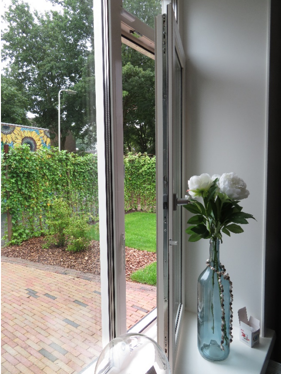
Figure A34. New windows, with extension showing depth of wall
