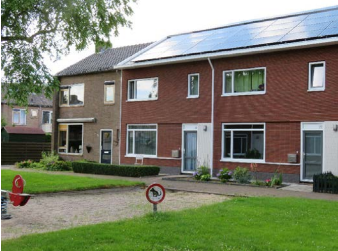
Figure 36. Residents did not approve the work in the end unit (left)
