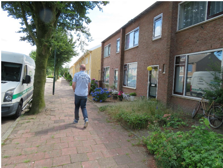
Figure A38. Building not yet renovated
