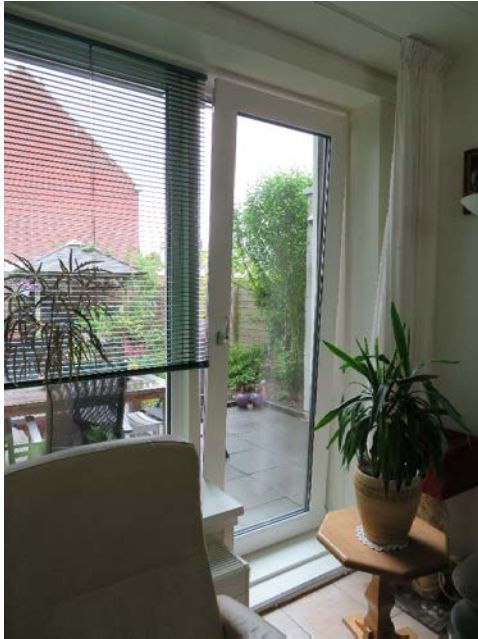
Figure 18. Doors and windows frequently can tilt in to provide added ventilation.
