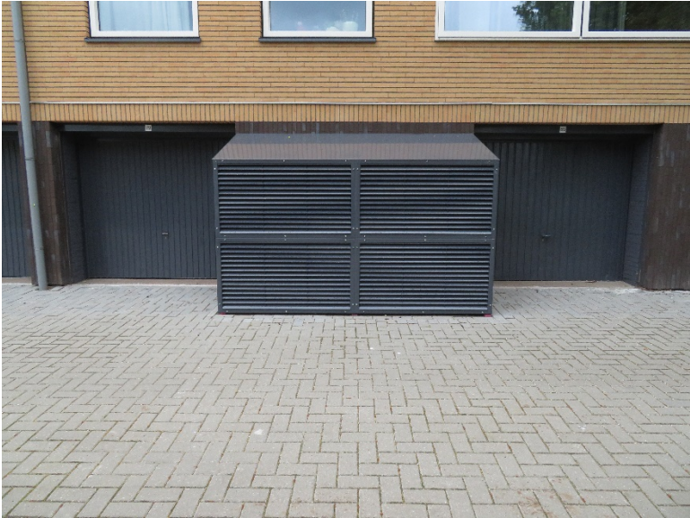
Figure A25. Exterior mechanical shed attached to renovated building
