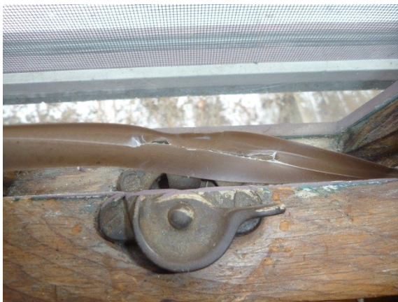
Figure 4: V-strip Failure
