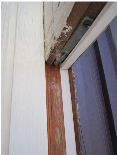
Figure 2: Plastic V-strips Installed
