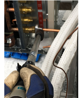
Torque wrench application
