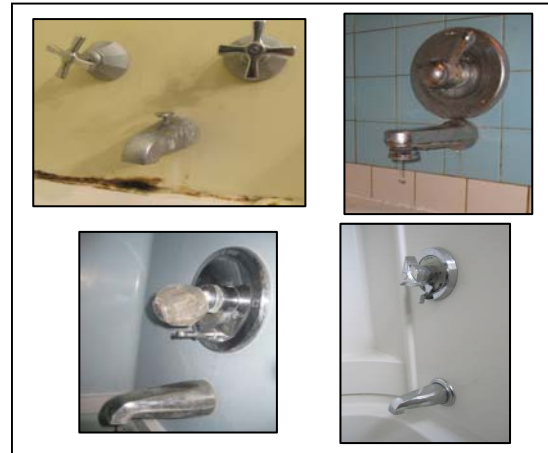
Figure 2: Examples of plate diverters. Clockwise from upper left: a lift on the tub spout diverter with a two-handle valve; a pull-down ring on the tub spout diverter with a single-handle valve; a sliding lever on the valve plate with a single-handle valve; and a button on the valve plate with a single-handle valve.
