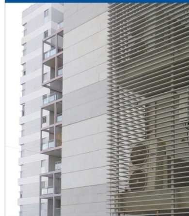
FIGURE 1 Air-source heat pumps.
