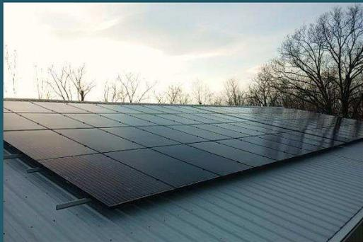
This **21 kW solar photovoltaic system** was mounted on a barn near the clients home. Lines to connect the system from the barn to the house are buried underground. Our crew was **able to put up all 84 modules in a single day.**
